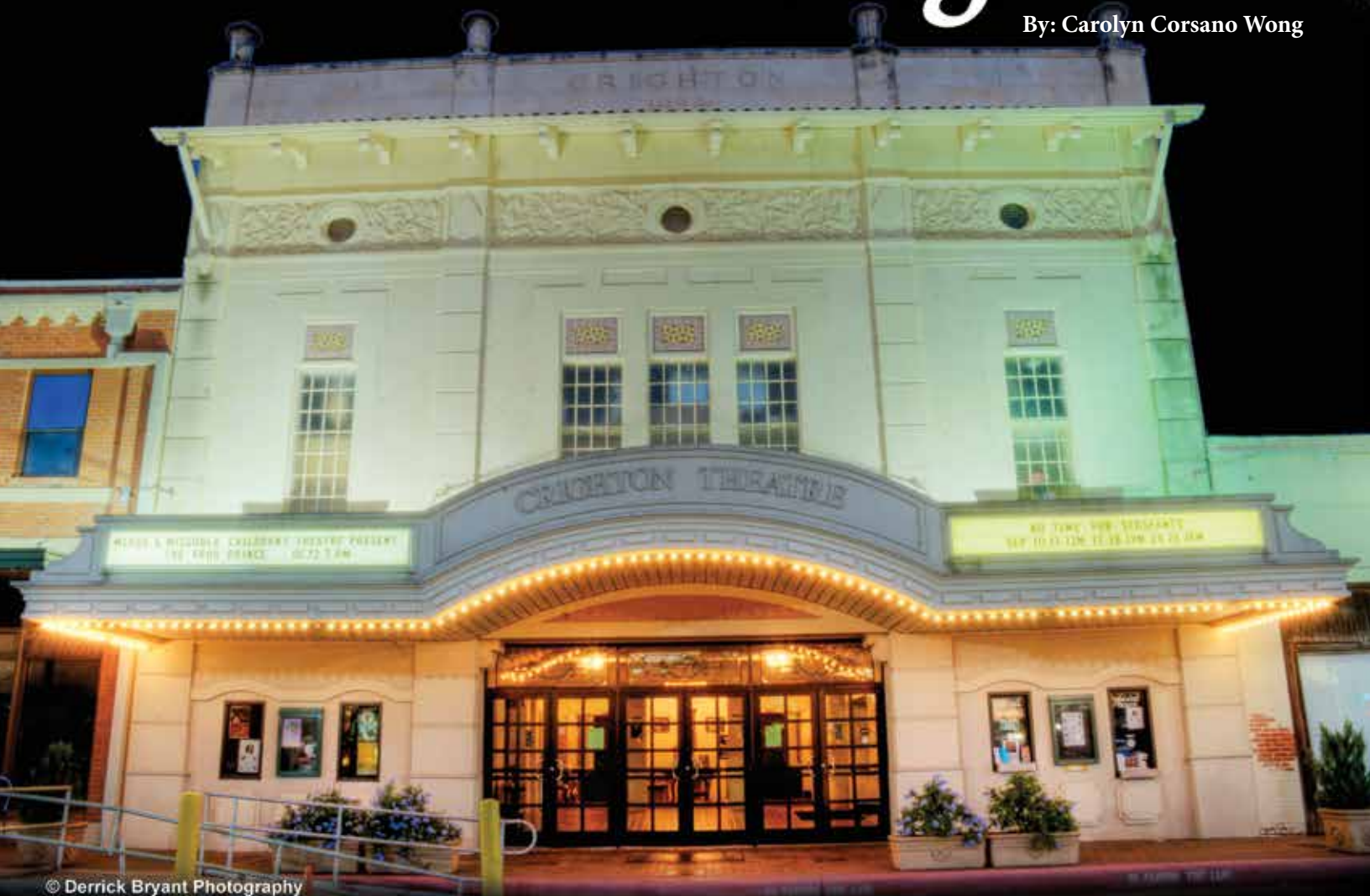
© Derrick Bryant Photography
